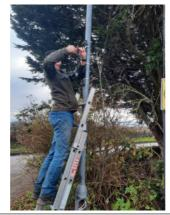
Paul Blackmore repairs the fault on the light and speed sensor on the Nassington Road, water had fused the setup, hopefully now rectified so won't happen again.
