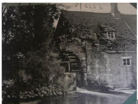
Flour was produced at Conegar for a number of years, but sadly, due to high maintenance costs and mill wright charges, things began to deteriorate. A few years into the 20<sup>th</sup> century the mill stone ceased to turn and what had been a good little 'undershot water mill' was lost forever.
